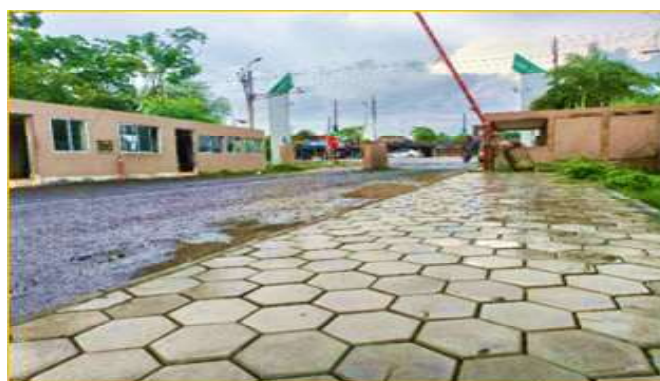
Picture 2.0: Laid Pavement Blocks at CLC Gate-03
